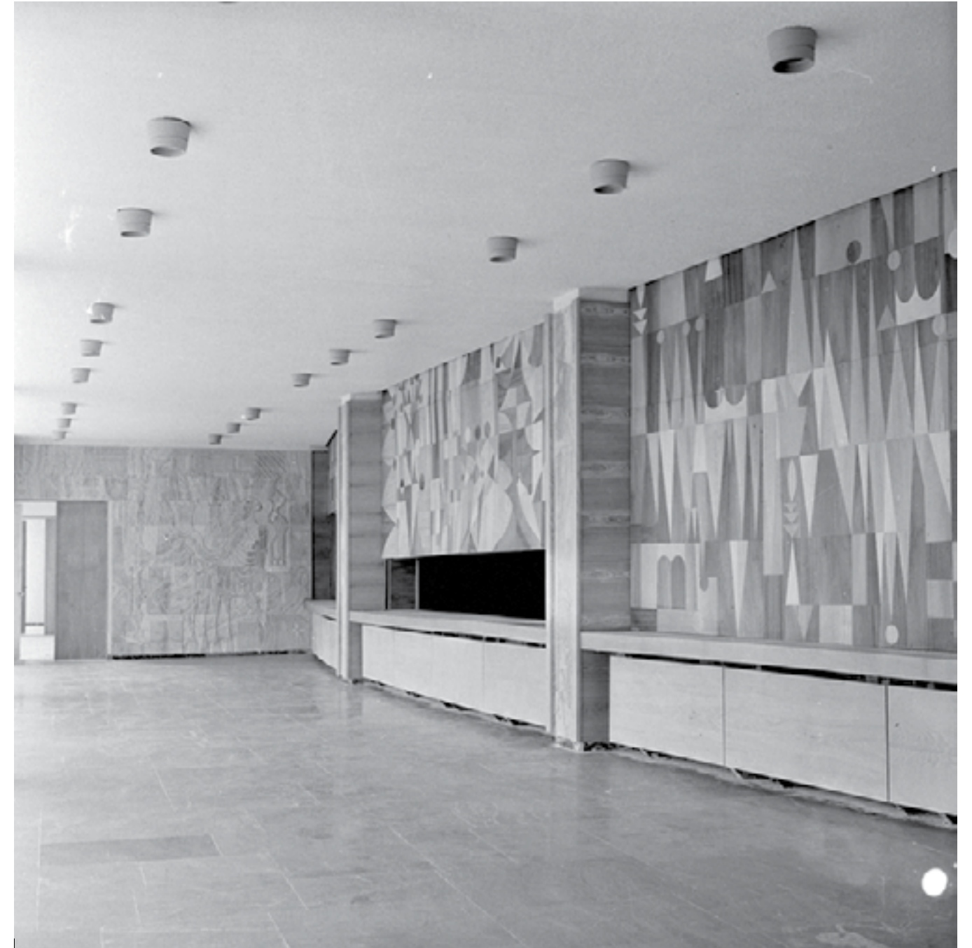
Vertically Sliding Marquetry Panels of the Main Hall Photo: Private Archive of Germane Ghudushauri
