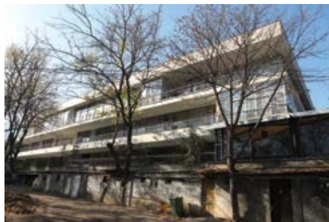
East Facade. 2016 Photo: Gogita Bukhaidze
