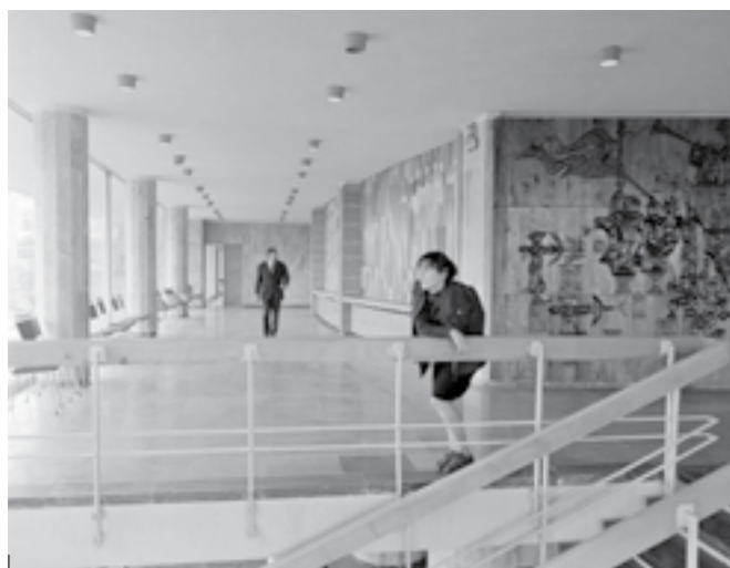
Staircase on the north-east of the building before demolition Photo: Germane Ghudushauri Private Archive
