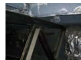
Figs. 17 and 18 Leaching in ribbed prefabricated concrete tiles arranged on metal trusses
