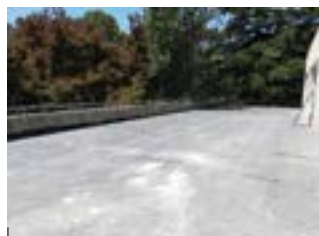
Fig. 7. View to the roof terrace
