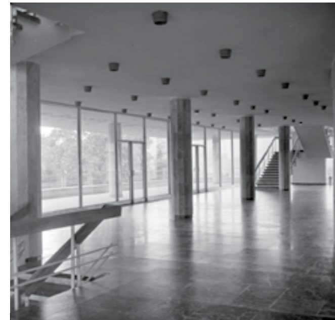
Northern Gallery of the first floor before alterations Photo: Private Archive of Germane Ghudushauri
