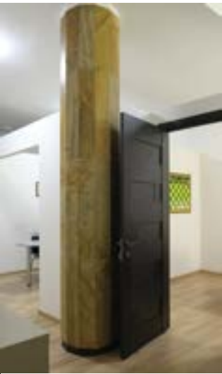
Tuff tile cladding of the column covered with the layer of varnish. 2018
