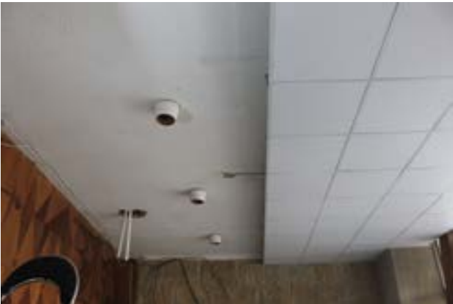
Process of Arrangement of Dropped Ceiling. 2018
