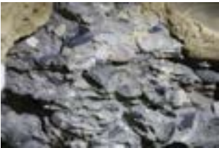
fig. 2. Sampling area, basement, bearing construction, close up
