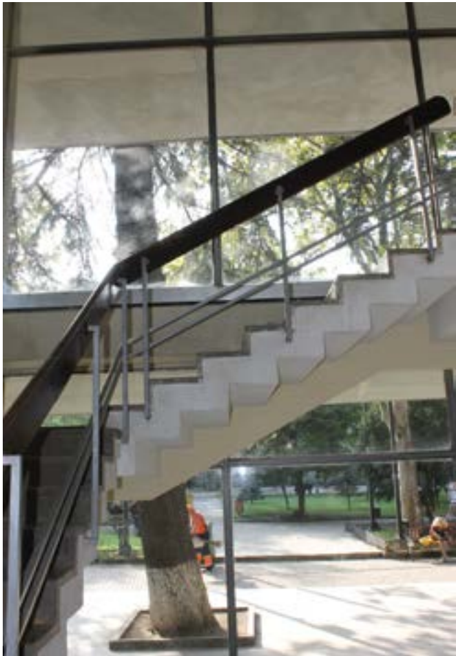
A Staircase in the Administrative Zone. 2019
