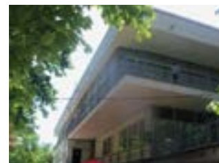
Fig. 2. The building as it looks today
