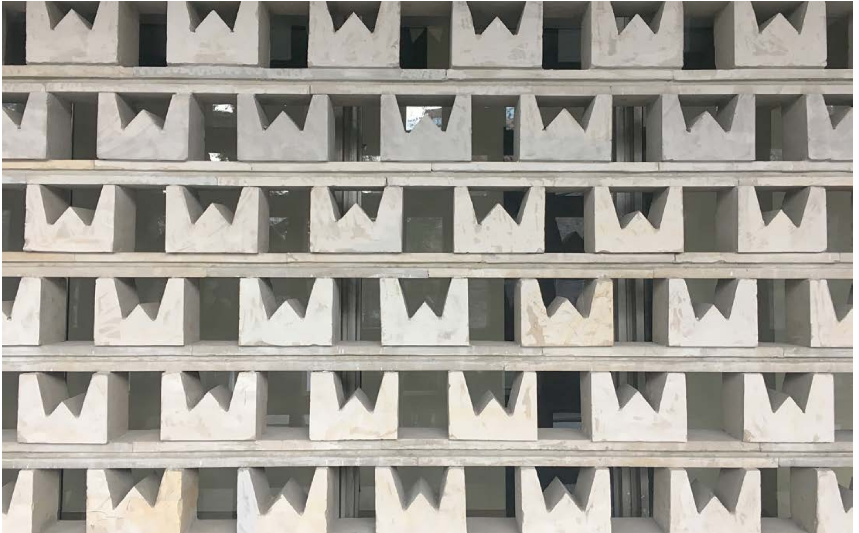
Decorative Stone Wall on the West Façade
