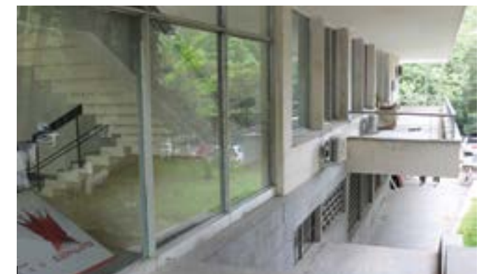
Cantilever balcony and aluminum vitrage. 2019
