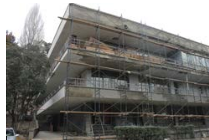
Process of replacing stone cladding on east façade. 2018
