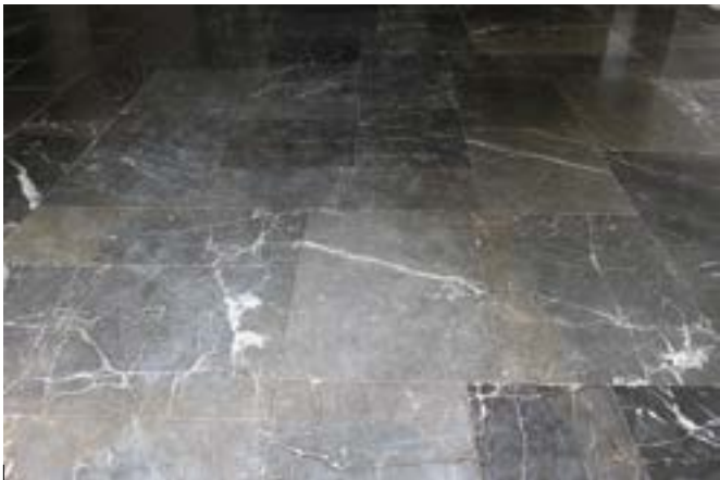
Sadakhlo Marble Tiles of regular Shape and Size Used as Flooring. Vestibule. 2018
