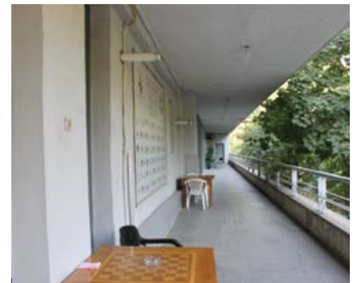
Balcony on East Façade. 2018
