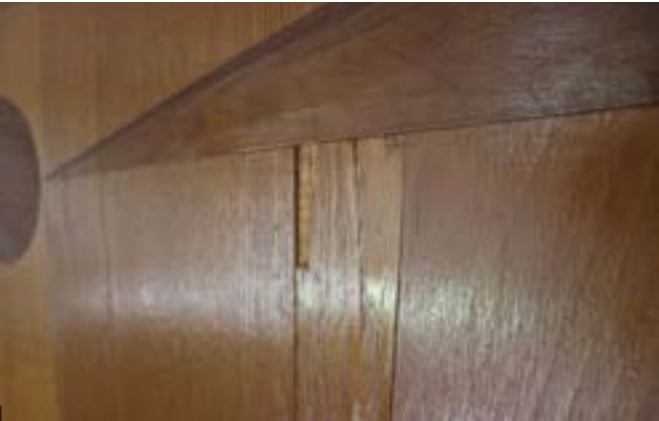
Surface Damage on Vertically Slidable Marquetry Panels
