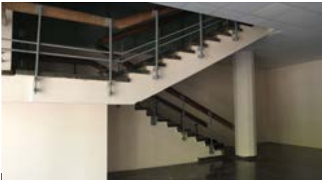
Staircase in the northwest of the interior. 2020
