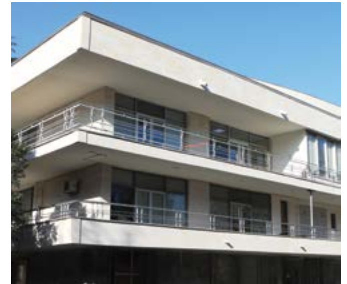
Renewed Stone Cladding on the East Façade.
