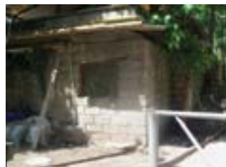
Fig. 4 Recent addition at the basement level
