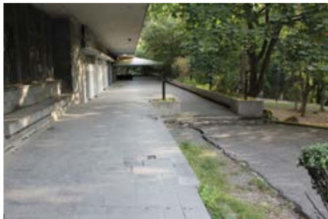
A Terrace on the Basement Floor. East Side of the Building. 2018
