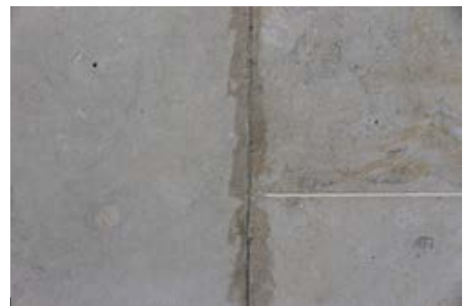
Replaced stone cladding of the façade in 2018.
