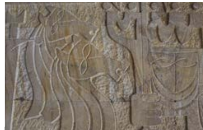
Detail of the wall faced with artistically processed stone slabs. 2020
