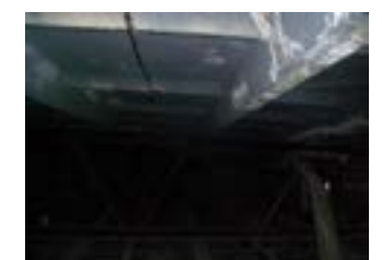
Figs. 17 and 18 Leaching in ribbed prefabricated concrete tiles arranged on metal trusses
